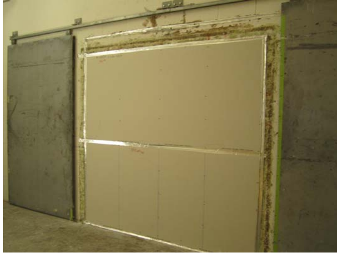
Figure 3: Photograph of receiver room sheeting layer
