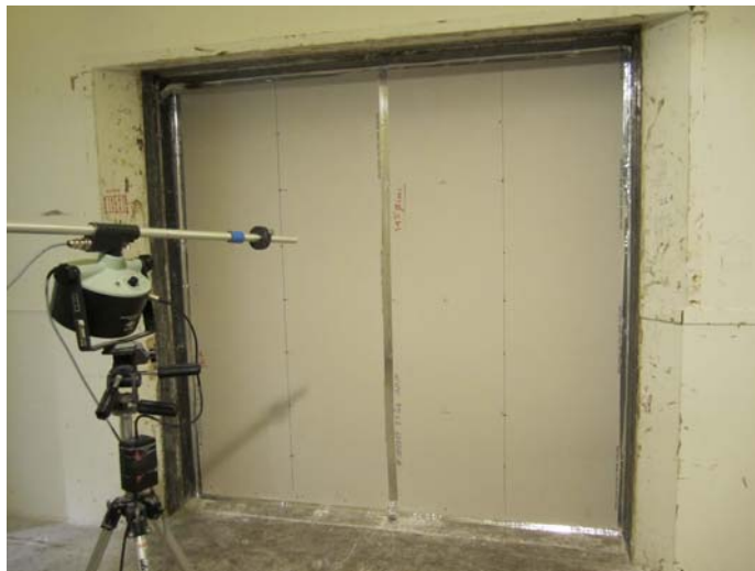
Figure 2: Photograph of sealed source room sheeting layer
